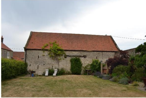
Barn 2 – South Elevation
