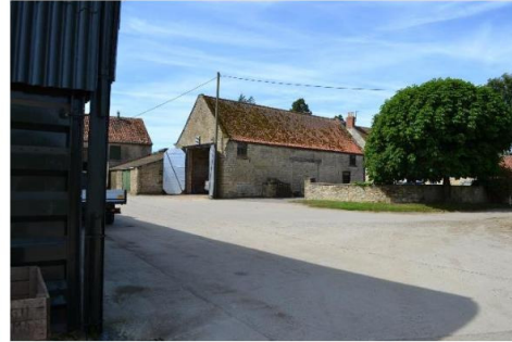
Barn 2 – Rear Elevation
